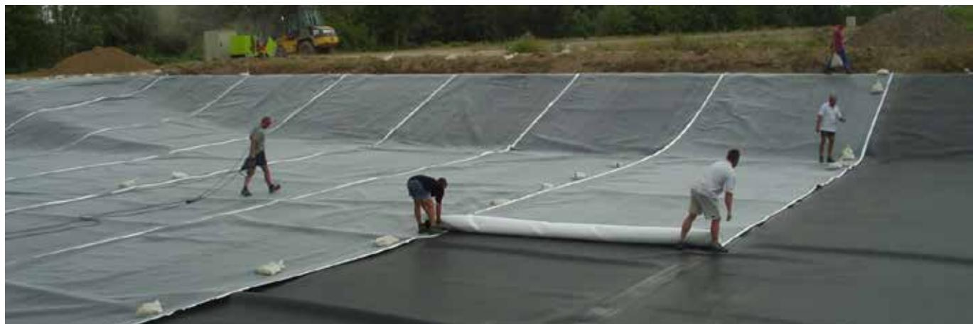
HDPE geomembranes act as a seal for central ground filters that collect rain water from flight operation areas with contamination from surface de-icing.
