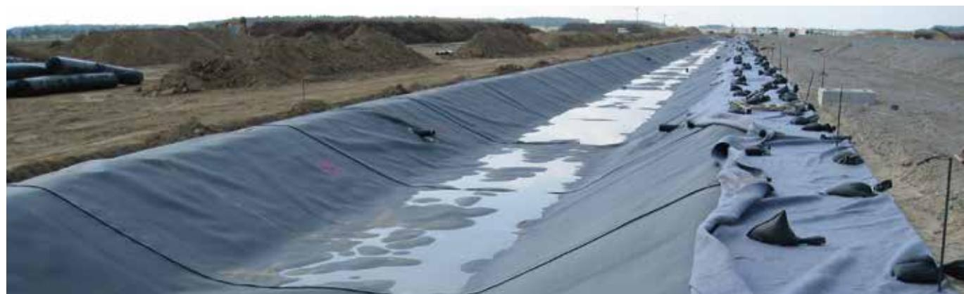
Local ground filters are also being made from HDPE geomembranes to go next to the runways and taxiways. These are being used to treat rainwater with impurities from flight operations and surface de-icing before it is transferred to the central ground filters.
